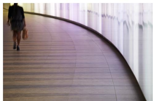
Additionally, the floor tiles needed to be over 1200mm wide, to modulate with the faceted LED lightwall. Craven Dunnill sourced the high quality, Italian-made tiles which are unglazed, rectified and are PTV 40+. In addition, floor tiles were supplied for the escalator hall and steps.
